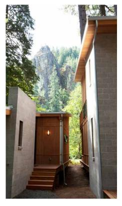
Clad in wood panel and batten siding, the dry zones include the living room, dining room and bedrooms. Resting on steelreinforced concrete piers, these spaces appear to float above the ground, creating a sense of lightness as the landscape flows beneath. Unlike conventional foundations, these concrete piers pose no harm to the roots of the surrounding Douglas fir trees.
